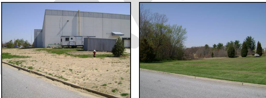
Figure 12: Commercial Sites for BMP installation (Photo Credits: Greg Rusciano)
