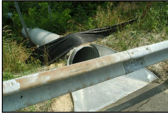
Figure 9: Stormwater conduit on Marl Run
